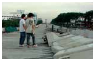
Kelana-Subang Elevated Highway Link
